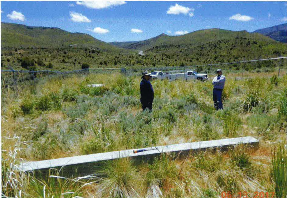
Looking south with cut-off headwall in foreground
