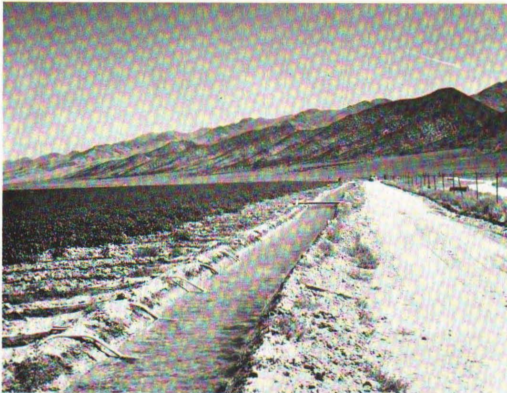
Photograph 4. View north in T. 21 N., R. 54 E. showing main ditch, siphons and furrow irrigation of potato field.
