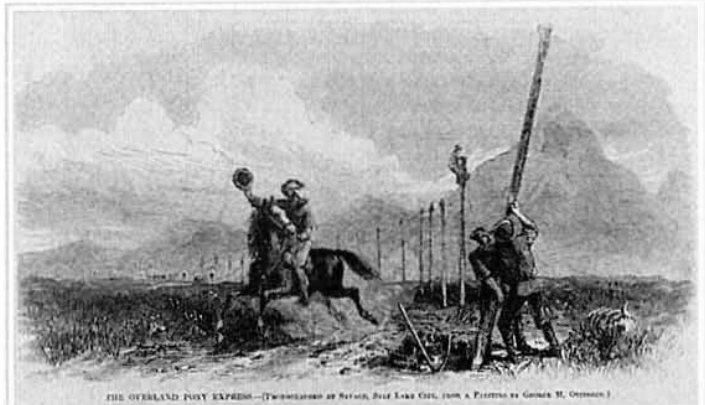
Wood engraving depiction of the construction of the first transcontinental telegraph, with a Pony Express rider passing below.
