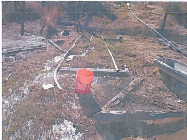
Additional outflow from R04233 via pipe.
