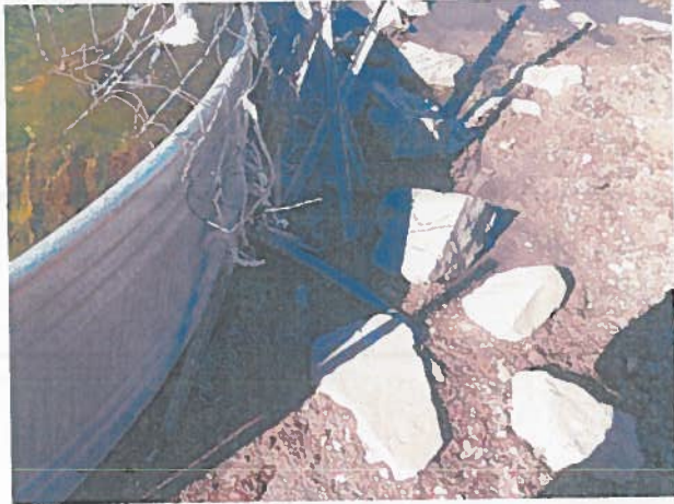
Inlet pipe, east side of stock tank. Location of spring source cannot be determined.
