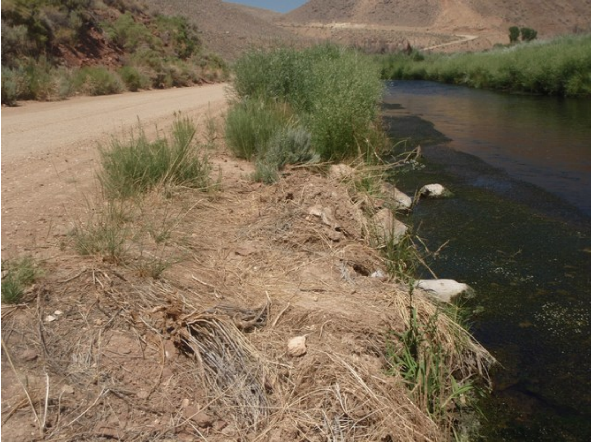
Figure 2.1-127. Side-cast pushed directly into the river.
