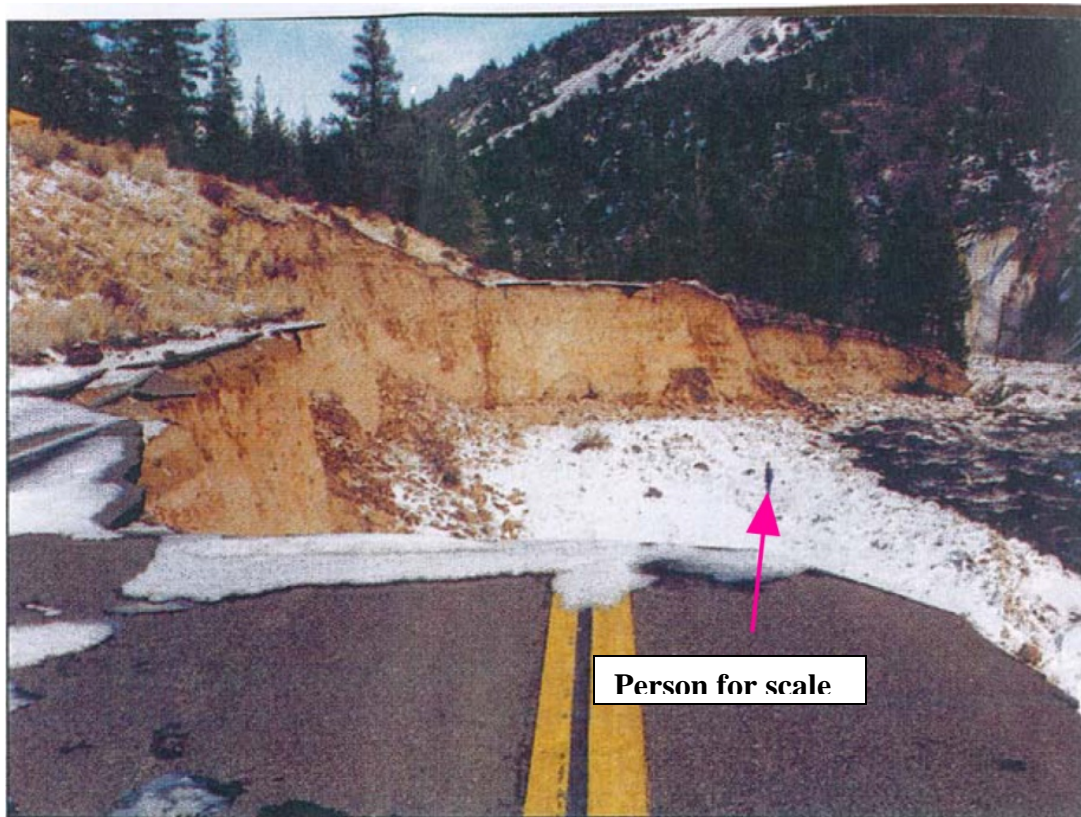
Figure 2.1-51. The photo illustrates the magnitude of erosion of the highway by the flood of 1997. Note the person for scale (from Schmidt, 1997).
