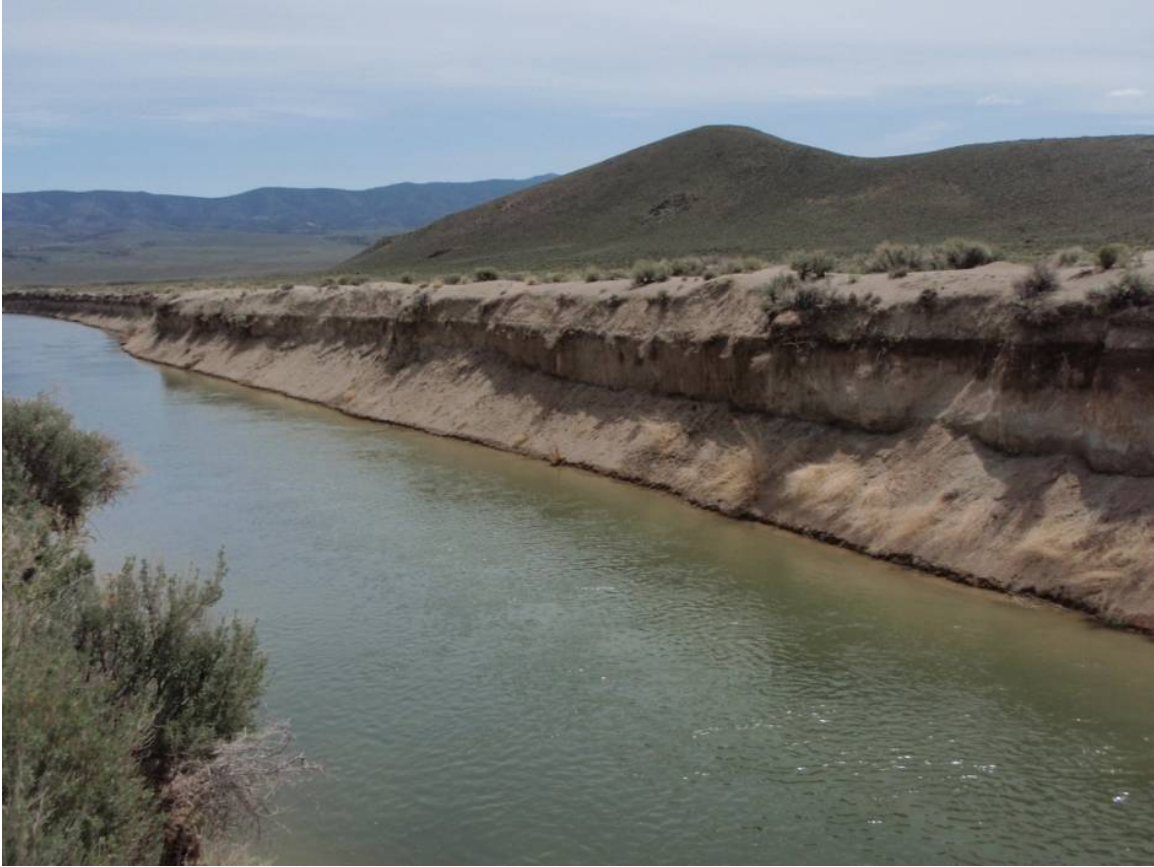
Figure 2.1-111. Over steepened banks on the Topaz return channel. These banks are approximately 20 ft high.
