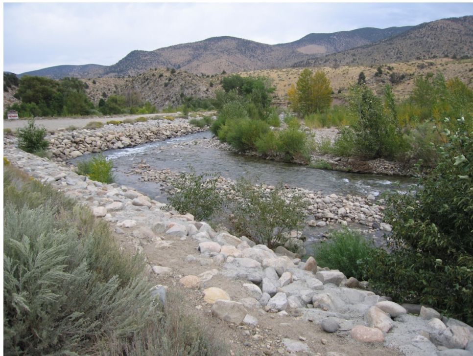
Figure 2.1-50. Riprap protecting highway and structures in modern times near the downstream end of WW3. The view is looking downstream.
