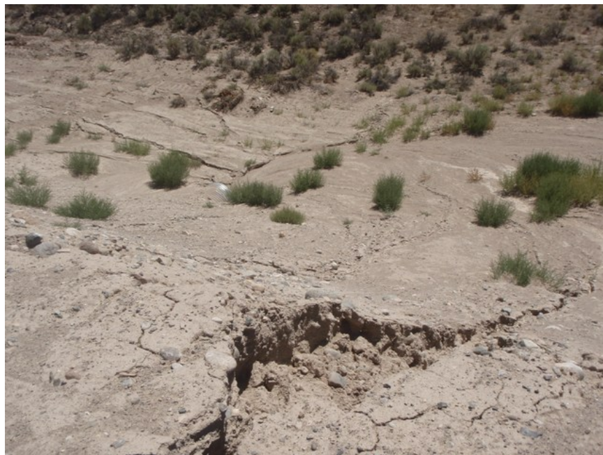
Figure 2.1-125. Sediment off of fill slope routed to culvert, no BMPs present.
