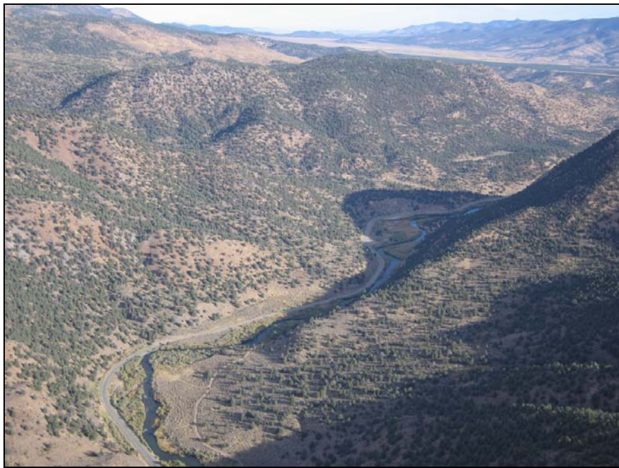
Figure 2.1-68. Aerial photograph of EW2 downstream of Bridgeport Reservoir as it flows through a relatively restrictive canyon. Flow is from the bottom to the top of the image.
