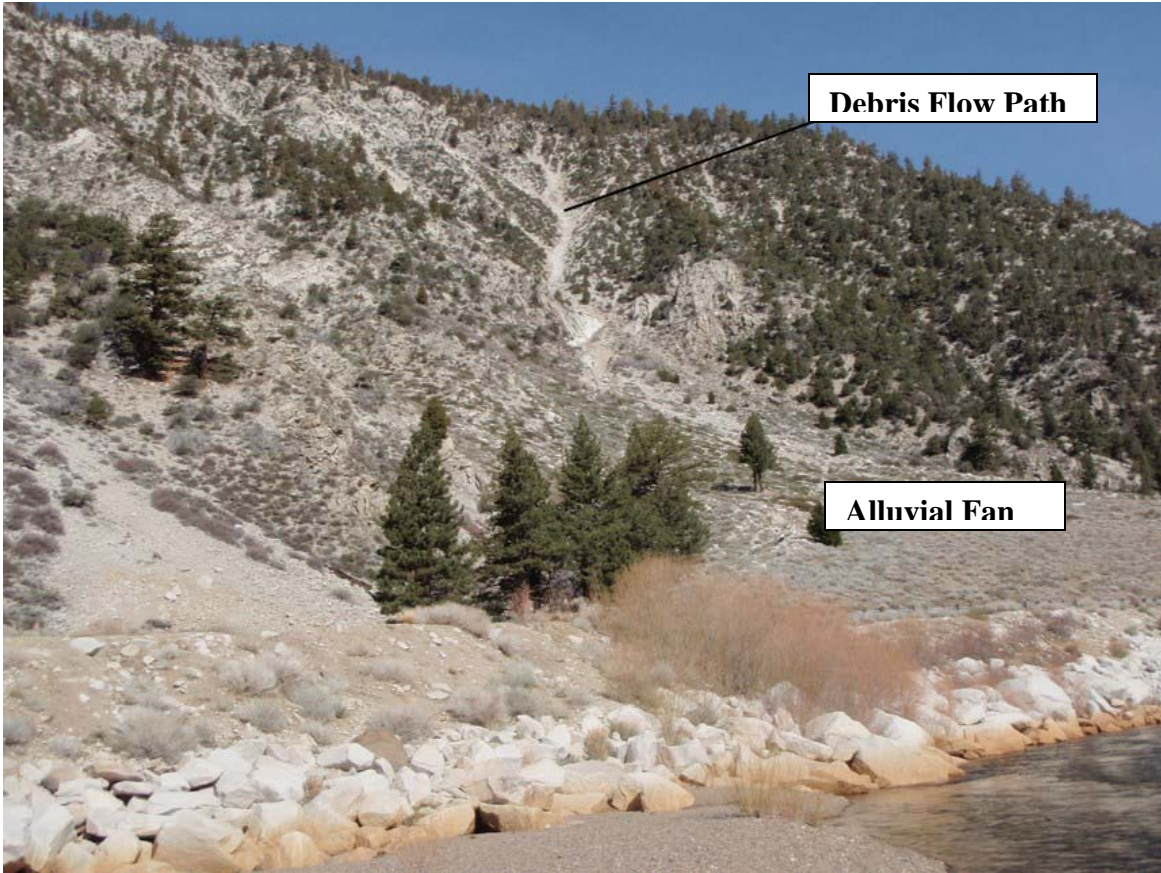
Figure 2.1-107. Debris flow path coming off the west side of the Walker Canyon just below Chris Flat.
