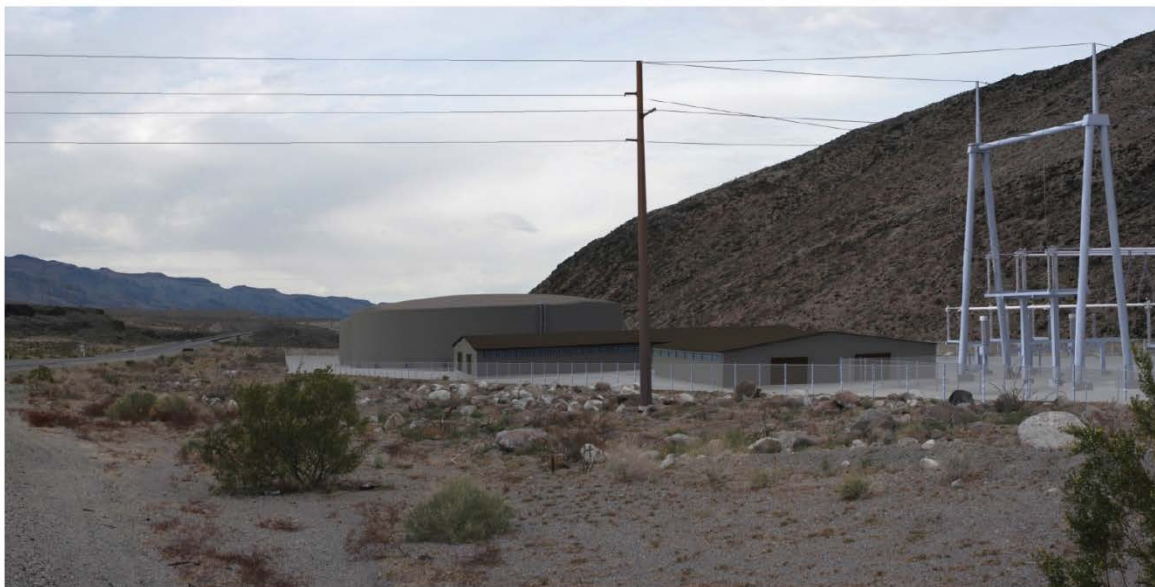
KOP 36 Photographic simulation of Coyote Spring Valley Pressure Reducing Station. Common to all alternatives.
