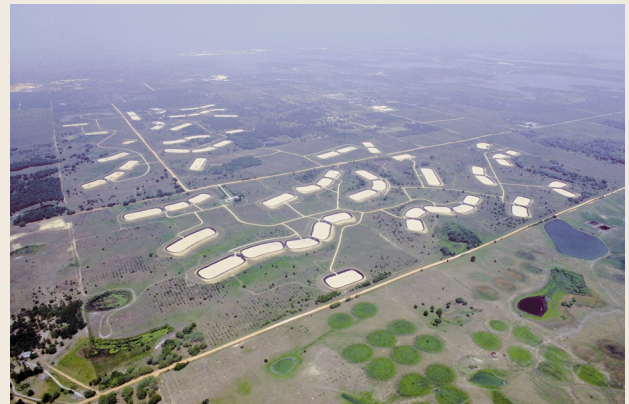
Rapid infiltration basins. (Photograph courtesy of Water Conserv II facility, Orlando, Florida.)
