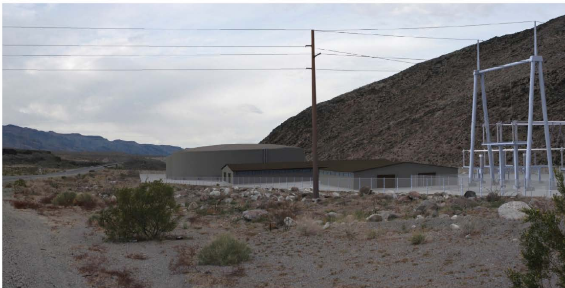
KOP 36 Photographic simulation of Coyote Spring Valley Pressure Reducing Station. Common to all alternatives.
