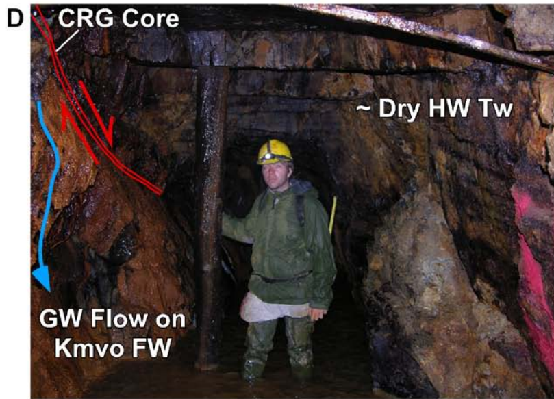
Figure 18.—Continued Photographs of the Standard fault vein from Levels 3 and 5 in the Standard Mine. (D) Asymmetric groundwater flow on the Ohio Creek footwall principal slip surface of the Standard fault vein in Level 5. Note the Wasatch hanging wall is nearly dry. (E) Detail view of groundwater flowing (blue arrows) on the tripe-like (orange-beige to ochre) and drapestone-like (blood-red) flowstone types on the Ohio Creek footwall principal slip surface of the Standard fault vein in Level 3. CRG, clay-rich gouge; HW, hanging wall; HWDZ, hanging wall damage zone; FW, footwall; FWDZ, footwall damage zone; GW, groundwater.
