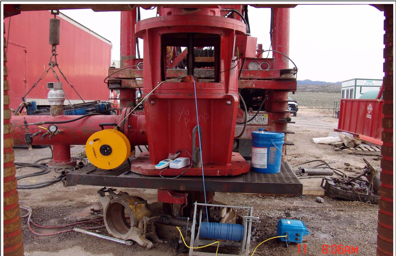
Figure A-3 184W101 Test Wellhead Equipment Setup
