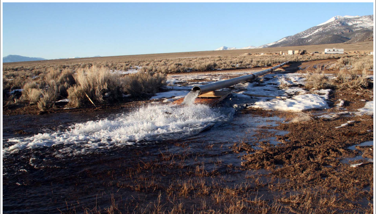
Figure A-4 Test Well SPR7007X Hydraulic Testing Discharge Line
