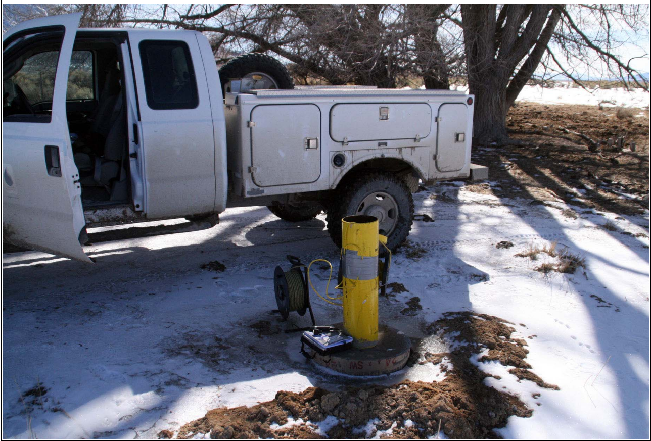
Figure A-8 Minerva Spring Piezometer (SPR7007Z) and Water Level Measurement Instrumentation
