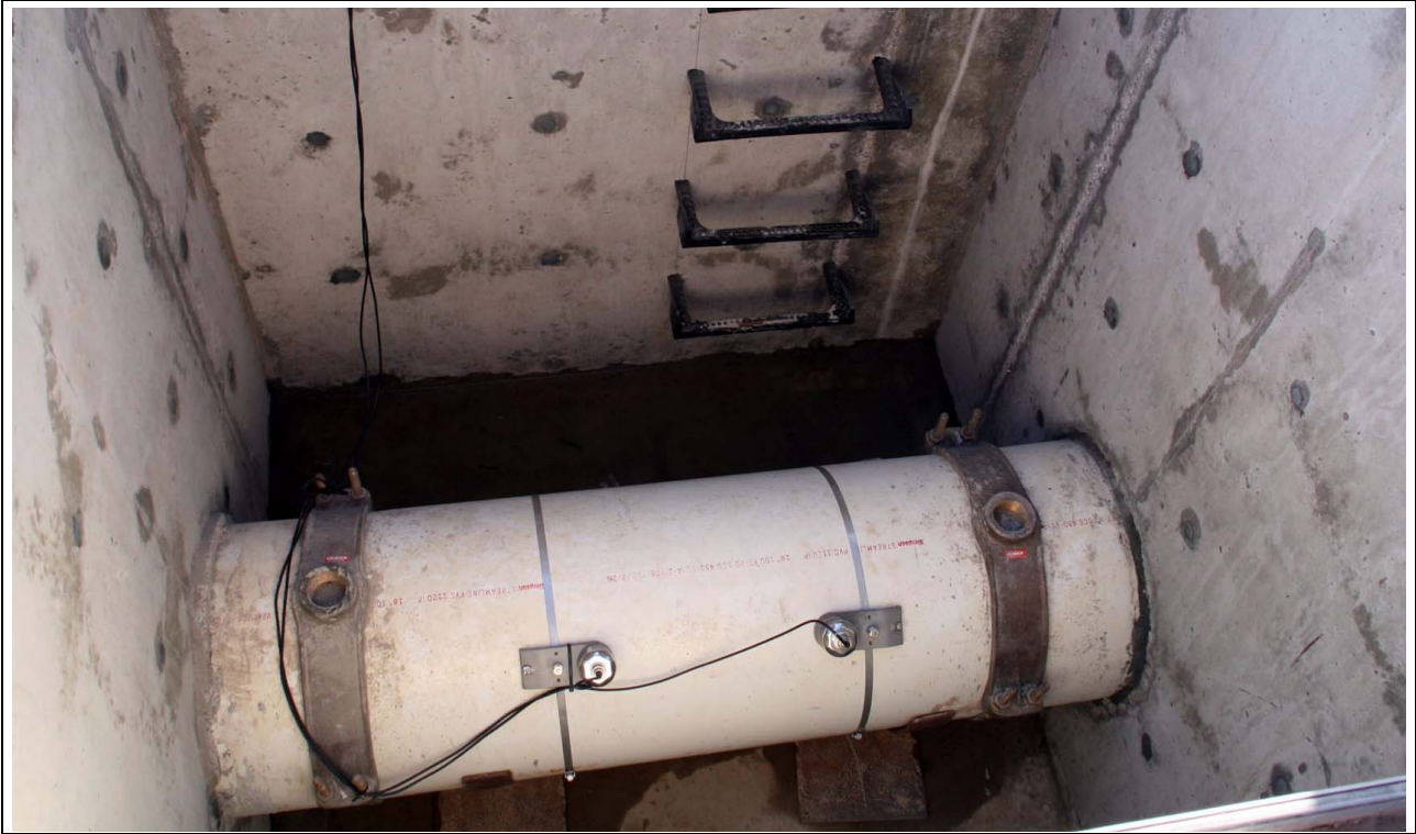
Figure E-8 Hiko Vault with Continuous Flow Meter on Hiko Discharge Pipeline, Summer 2009
