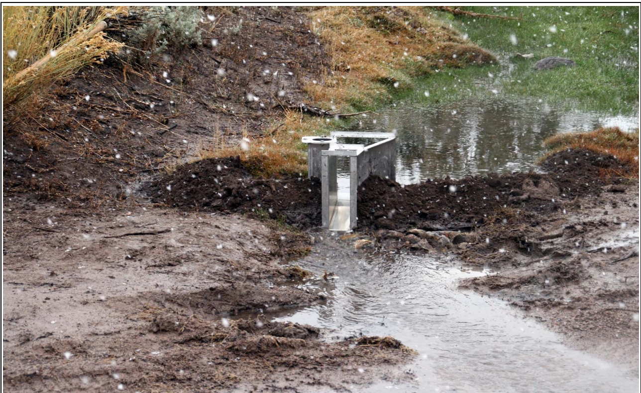
Figure E-18 Littlefield Spring Measurement Point, November 2010
