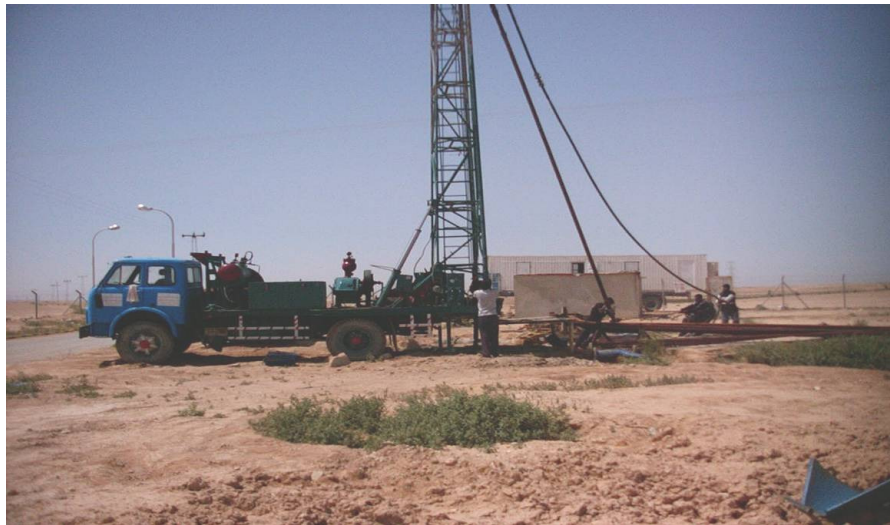
Figure H5: Rehabilitation of a water level monitoring well in AZB.
