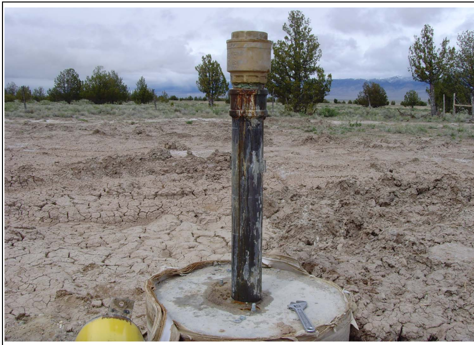
FIGURE 3 VIEW OF MONITOR WELL SPR7030M LOOKING NORTH
