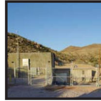
Municipal water source/ water treatment plant
