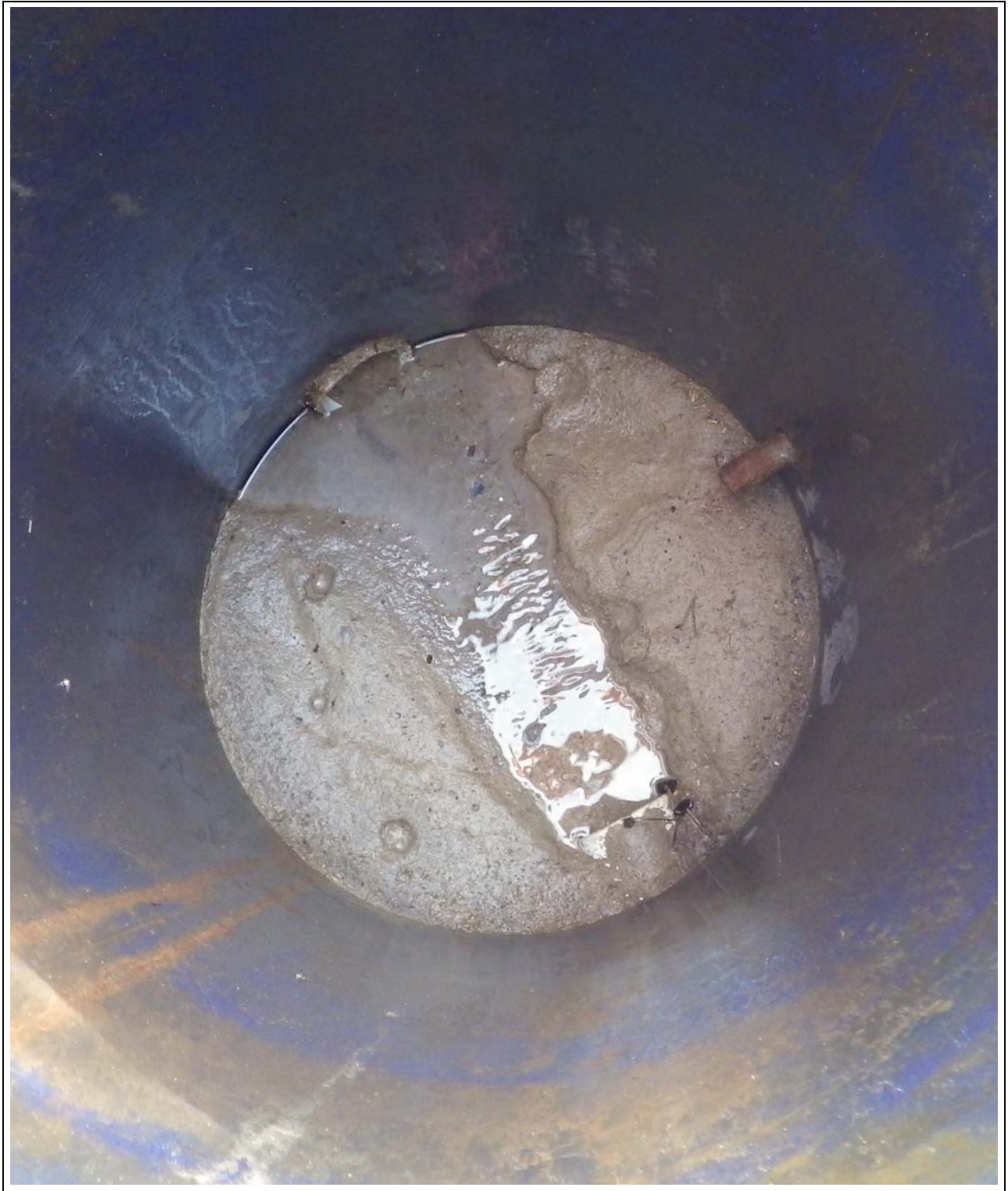
Figure E-10 Lewis Well Spring Collector Line Access Discharge, October 2013
