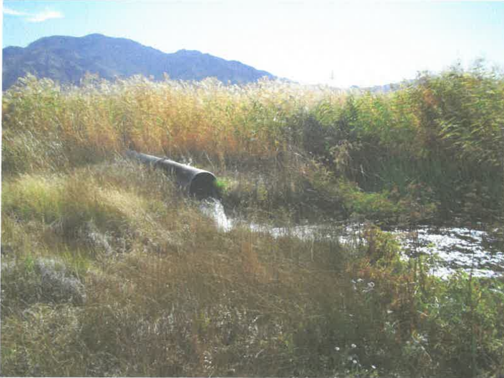
FIGURE 2. Looking upstream at the old “40ft culvert” on Sunnyside Creek. This culvert acted as a fish barrier to upstream movement and was removed in April 2015.
