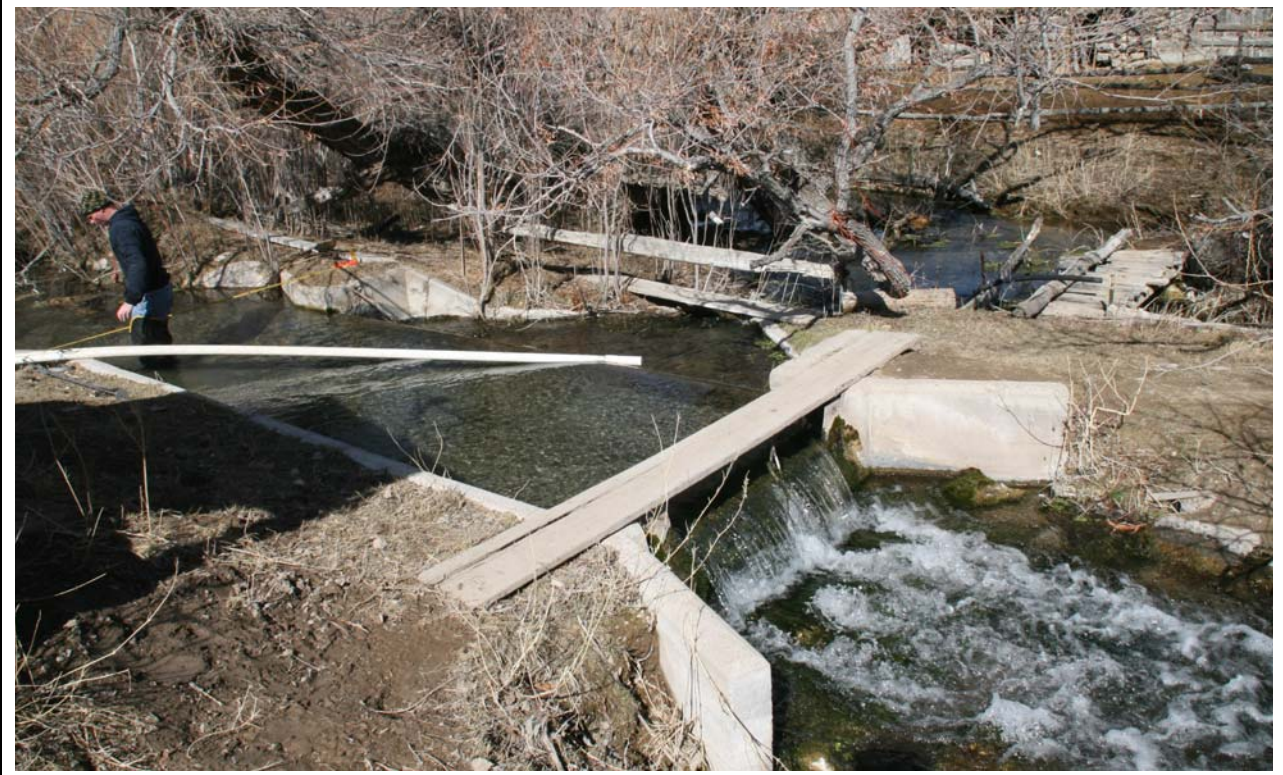
Figure D-1 Big Springs South Channel Weirs
