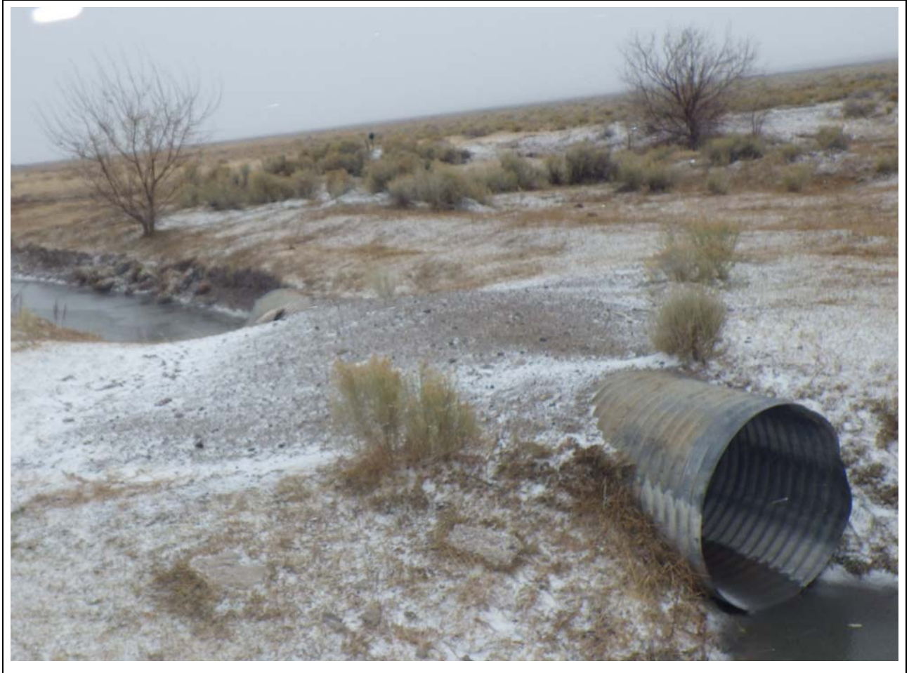
Figure D-9 High Line Diversion by Stateline Site 8.1
