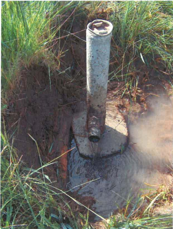
Figure 8. The wellhead from artesian well #4 that supplies water to the stockpond (June 25, 2014).
