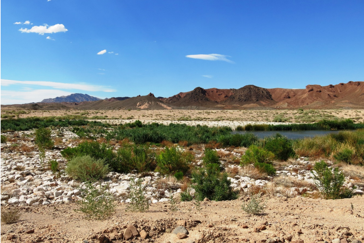
Figure 19. The Homestead Weir had nearly four and a half acres of vegetation established on it in 2015.
