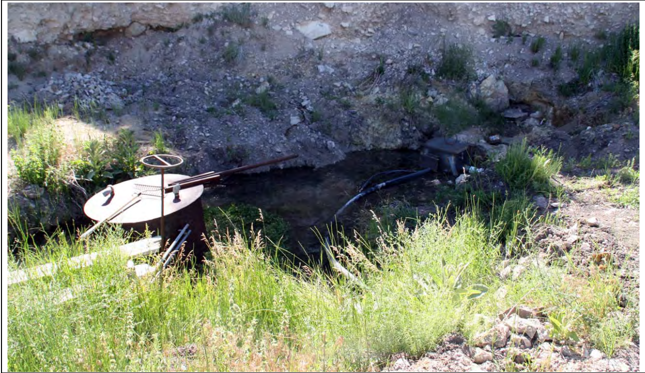
Figure 15-2 Turnley Spring Reservoir and Diversion Structure
