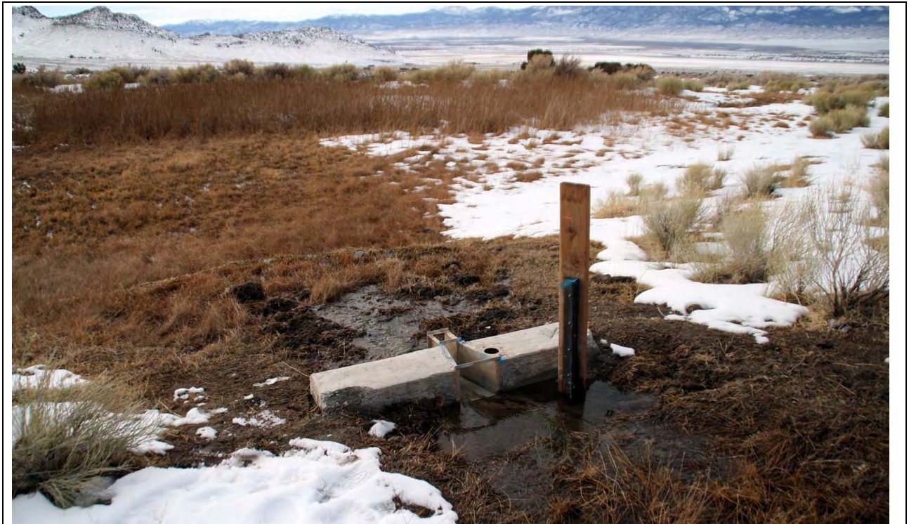
Figure 14-6 Rock Spring Flume
