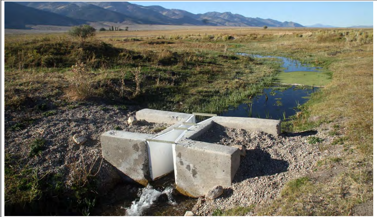
Figure 11-5 Keegan Springs Flume Located Southeast of Keegan Spring Nos. 1-3
