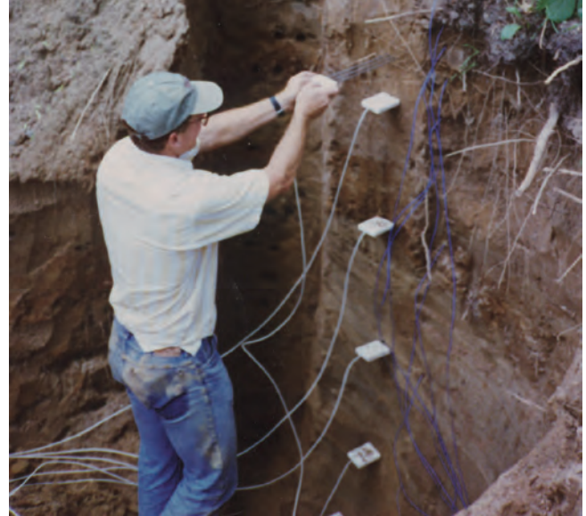
Installing moisture content sensors through the wall of a trench; the trench was later backfilled.
