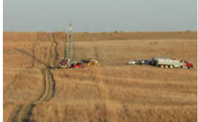
Installing an observation well.
