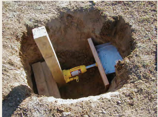
Installing pan lysimeter through trench wall with a hydraulic jack.
