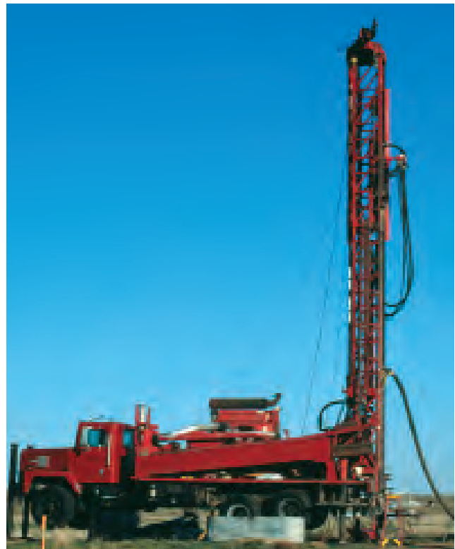
Well installation requires special equipment.
