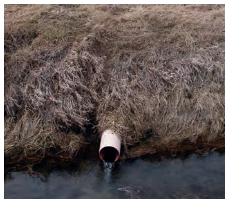
Tile drains are used to lower the water table in some agricultural fields.
