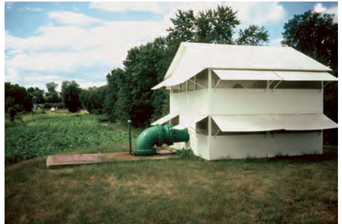
Pump house in northern Illinois.
