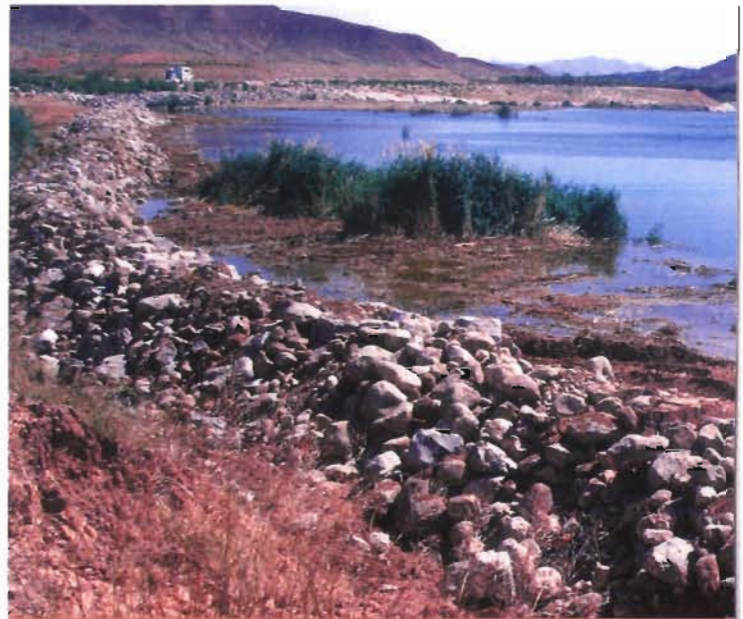
Bank stabilization is an important element to help deter erosion in the Wash. During 2005, an additional 4,400 lineal feet of bank protection was completed.
