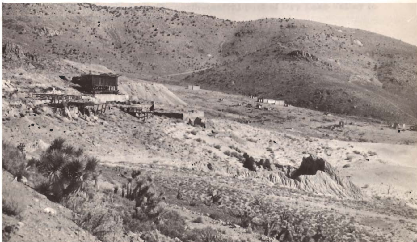
Photograph 4. View southeast of Delamar. Structure to left is remains of mill. Light colored band extending to right edge of picture is part of tailings. Wind action has heavily sculptured and removed a considerable volume of the tailings. In middle distance stone walls mark the principal area of Delamar townsite. Principal mining was in hill to left of left side of picture, although numerous prospect pits mark hill in background. Most of water supply for Delamar was brought in by pipeline from Meadow Valley Wash, 10 to 12 miles to the east.
