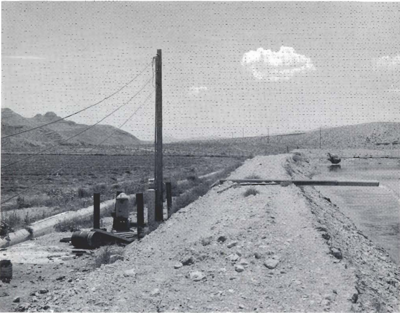
View of irrigation well 45/60-2a1, about 2½ miles north of Hiko Spring. Well is pumping an estimated 1,000 gallons a minute into reservoir from which water is carried in concrete lined ditches, one of which is shown at left of well, to field at left side of photograph.
