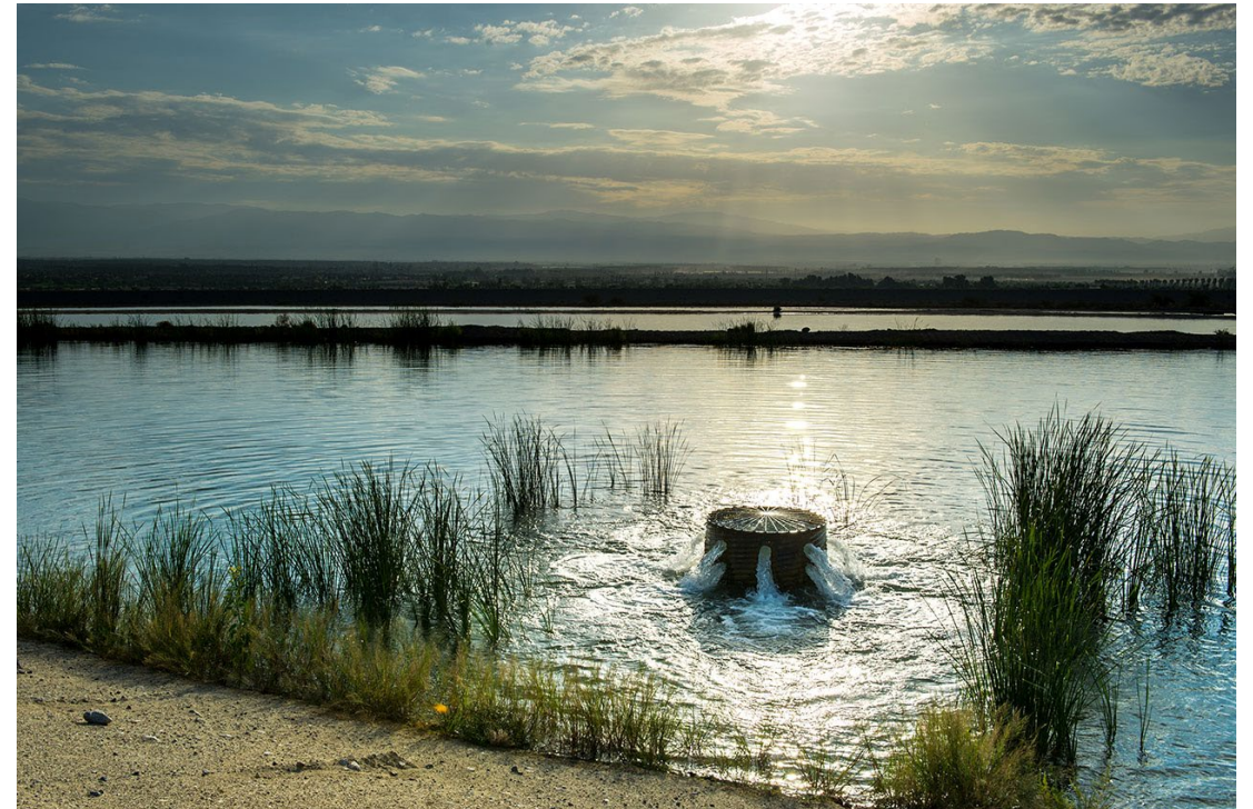
Photo of infiltration basin used for recharge of excess surface water
