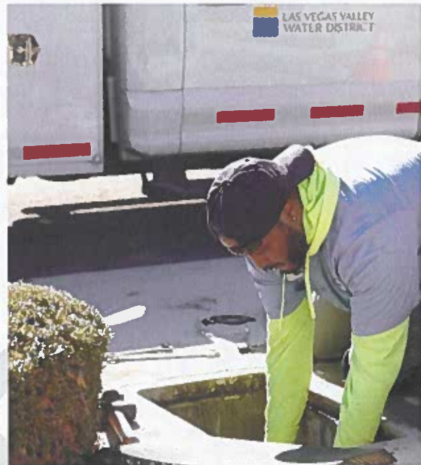
Photo: A field technician replaces a water meter.
